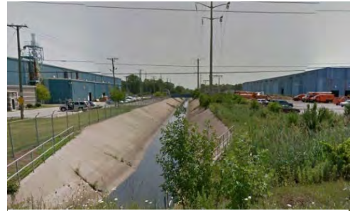
Figure 3.14-1 Google Street View – Calumet Union Drainage Ditch at Center Avenue (Harvey)
