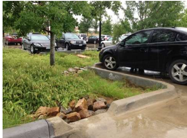
Figure 2 – Parking Lot with Bioretention
