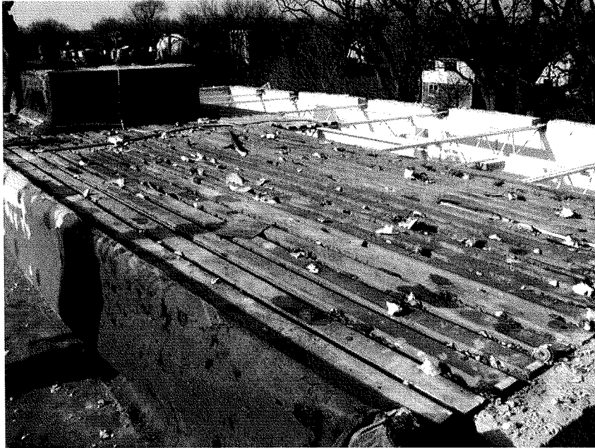
Lime Silo Room Roof Demolition
