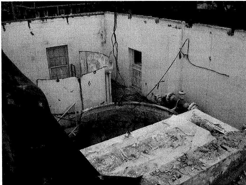
Lime Silo Room Silo Demolition Progress
