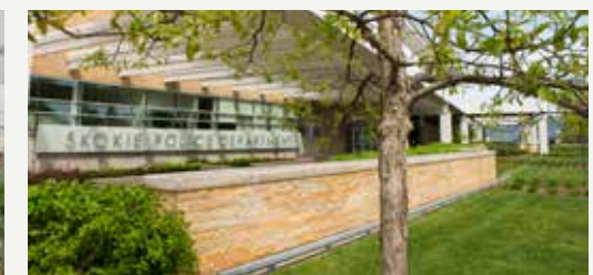
Skokie Police Station Headquarters can now retain 33,000 gallons of stormwater thanks to support from the MWRD.
