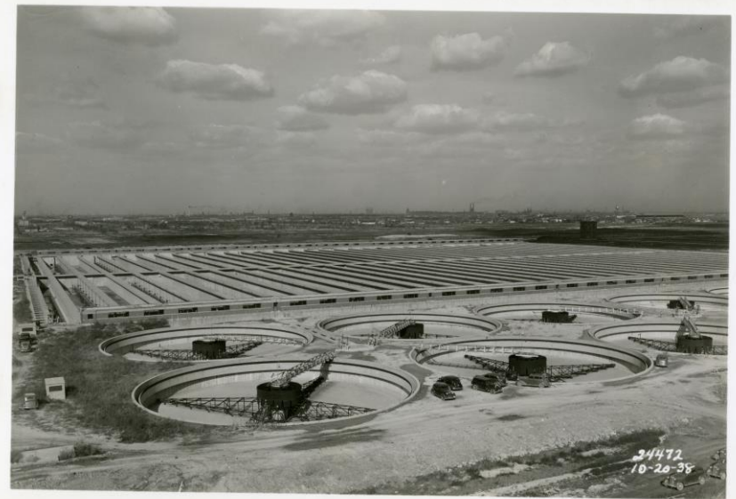
West Side Treatment Plant (Stickney) 1930
