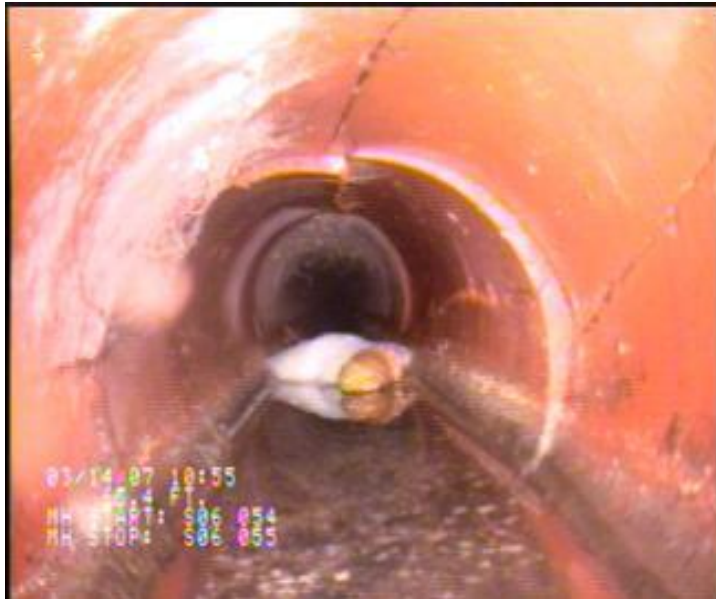
Before CIPP Lining
