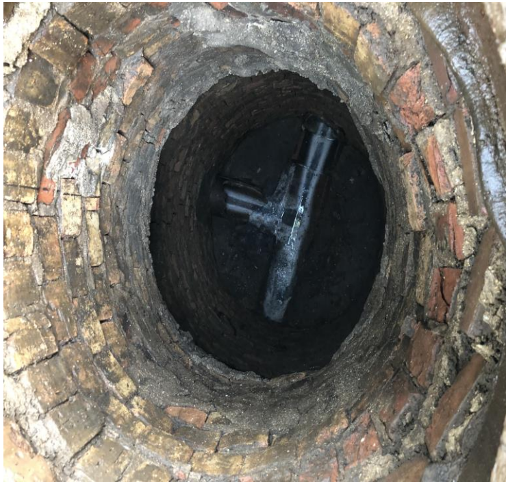
Existing Brick Manhole
