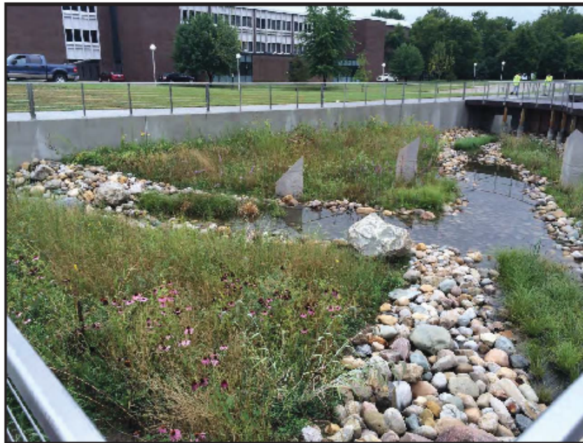
Figure 1.1. Constructed Wetland with river cobble channels and educational flood stage markers.
