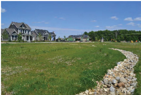
Figure 2.1.1 A Filter Strip Provides Pretreatment for an Infiltration Trench in a Residential Area
