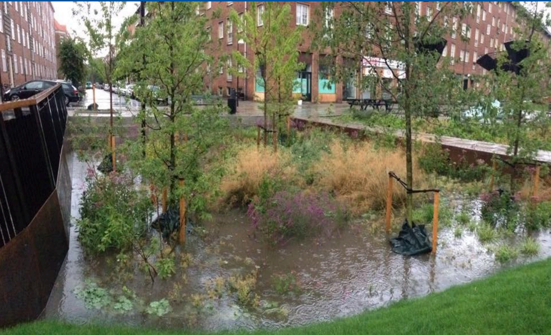
September 2015: Cloudburst event in Copenhagen, Denmark
