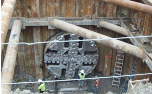
Entry to Junction Chamber 1
