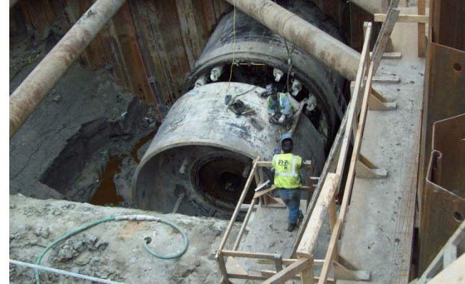
Split Sections in Junction Chamber 1
