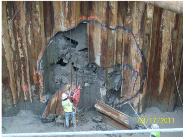
Entry to Junction Chamber 3
