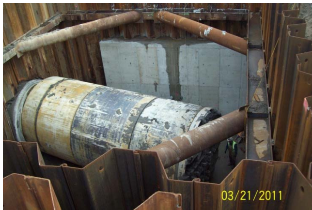
Turning TBM to E-W Alignment
