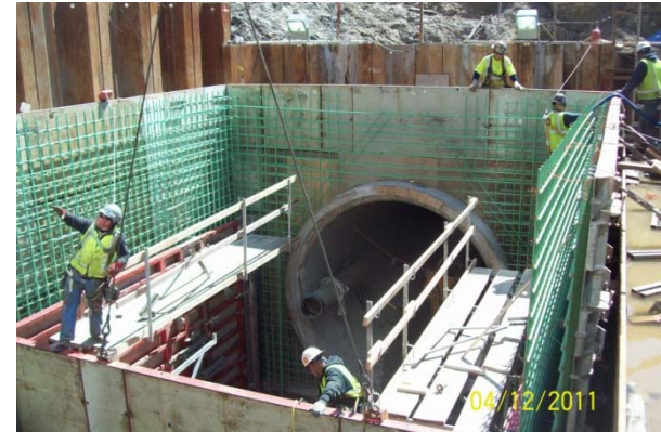
Wall Steel and Formwork
