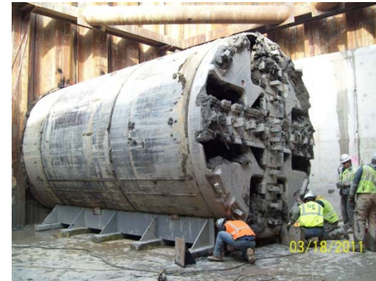
Drive TBM into Junction Chamber 3
