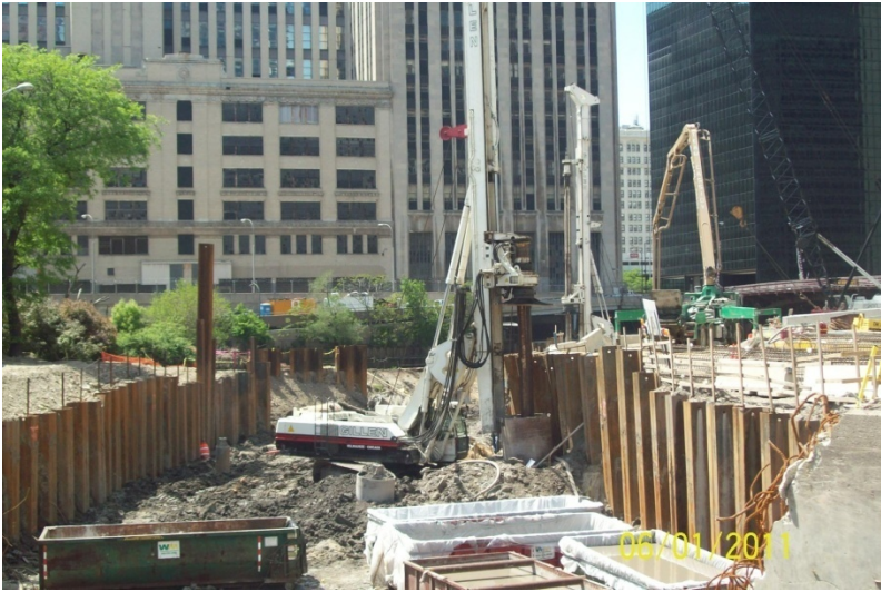
Tunnel E Caissons
