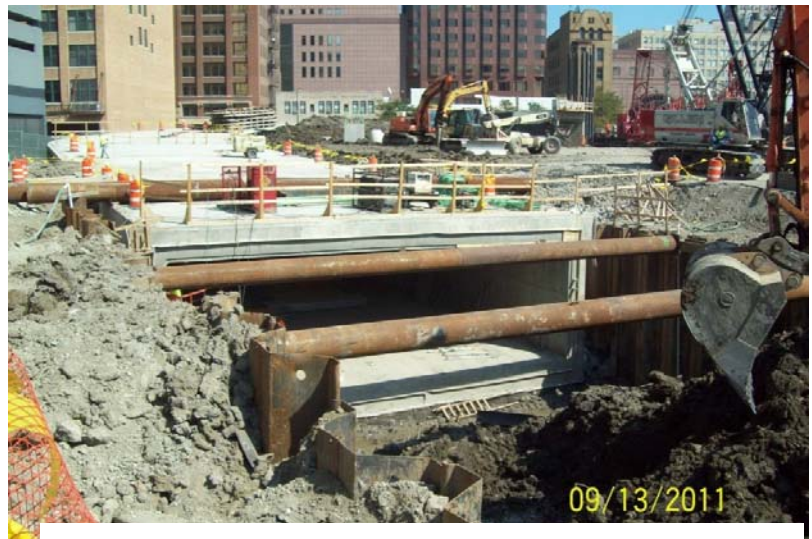
Tunnel E Excavation
