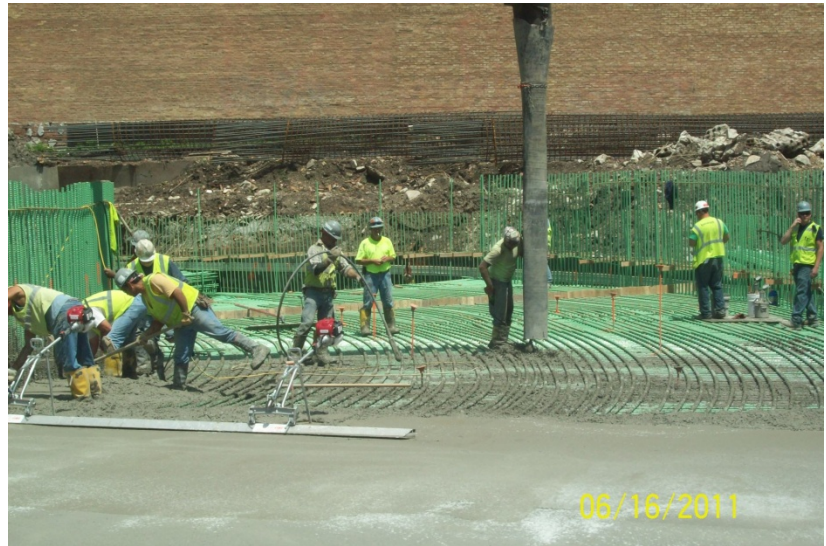
Tunnel E Base Slab
