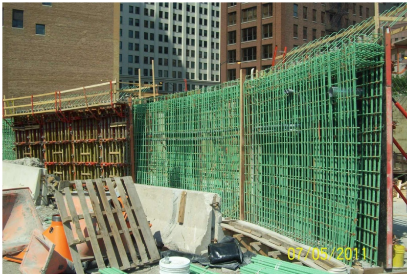
Tunnel E Framing Walls
