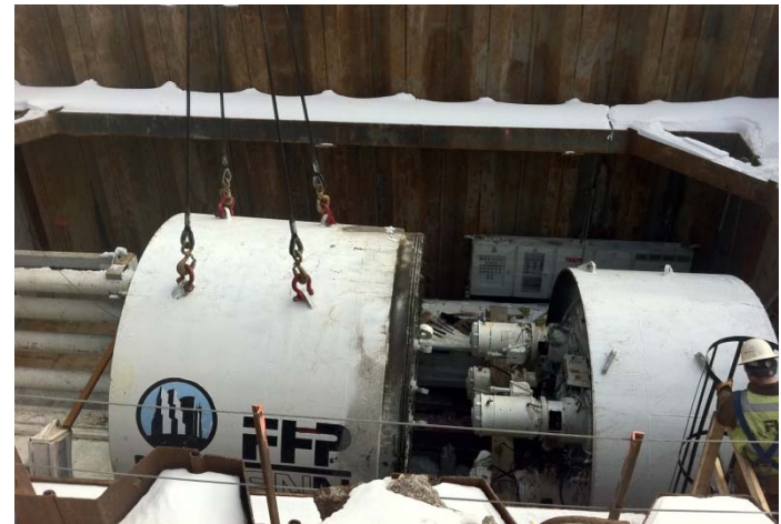
Middle TBM Section
