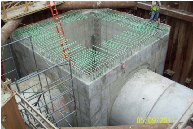
Stripped Junction Chamber
