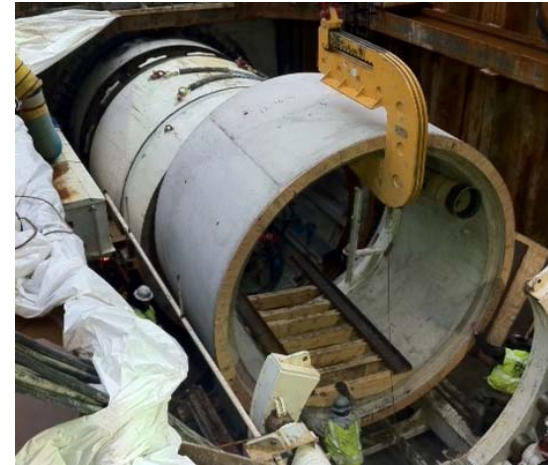
Setting Pipe Sections
