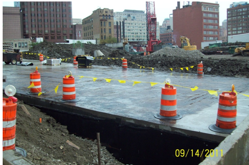
Tunnel E Waterproofing
