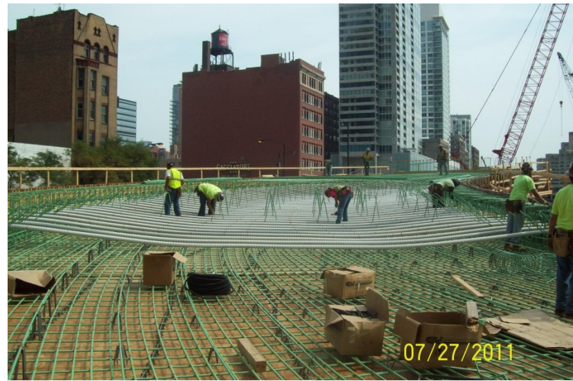
Tunnel E Roof Rebar and PT Installation
