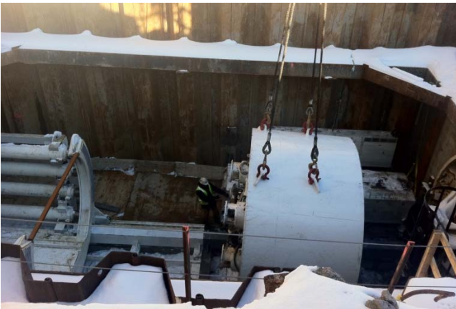
Lead TBM Section
