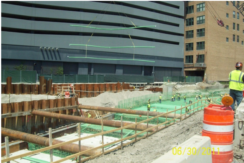
Tunnel E Rebar
