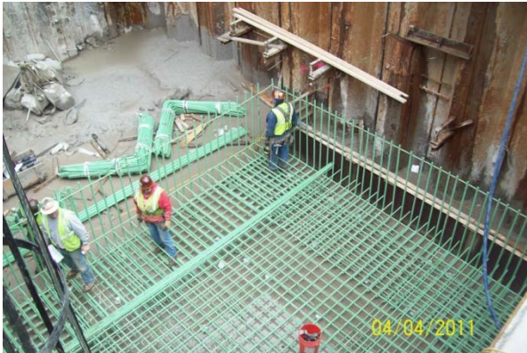
Base Slab in Junction Chamber
