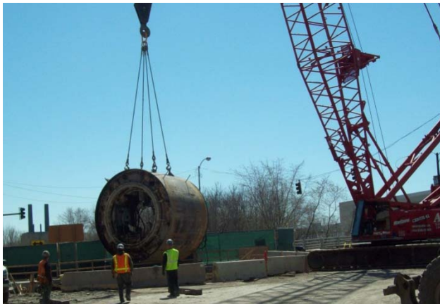
Extracting Equipment from Receiving Pit
