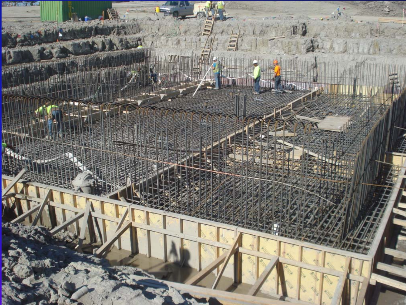
Concrete Base Slab
