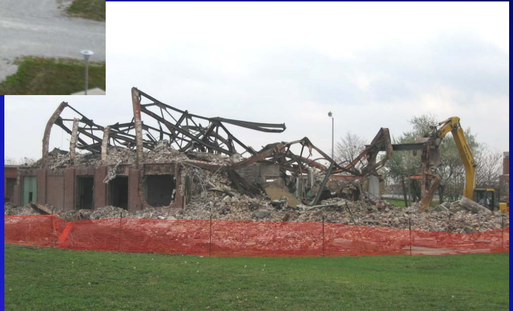
Demolition of Decommissioned Buildings
