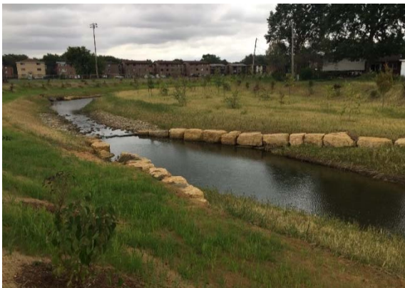
Streambank stabilization along Tinley Creek in Crestwood.
