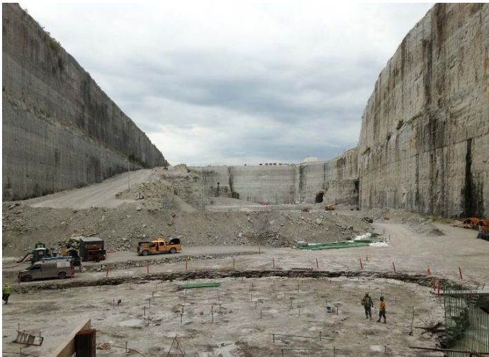
The first section of the McCook Reservoir, holding 3.5 billion gallons, is nearing completion in 2017. The reservoir is the final component of the Metropolitan Water Reclamation District of Greater Chicago’s Tunnel and Reservoir Plan.
