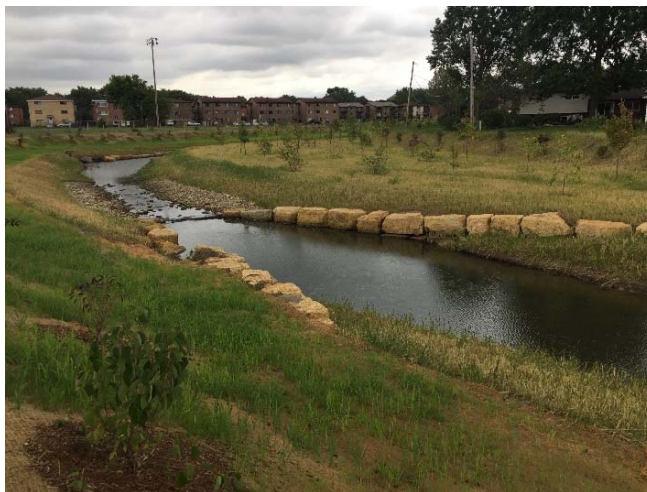
Flood Control and Streambank Stabilization Project on Tinley Creek in Crestwood.
