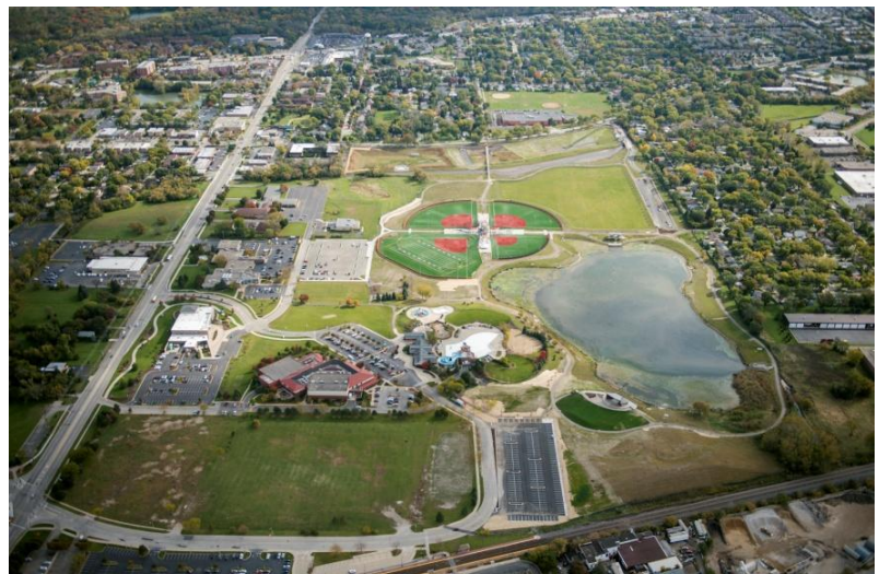
An aerial view of the Heritage Park Flood Control Facility, which was facilitated through an intergovernmental agreement between the District, the Wheeling Park District, and the Village of Wheeling.
