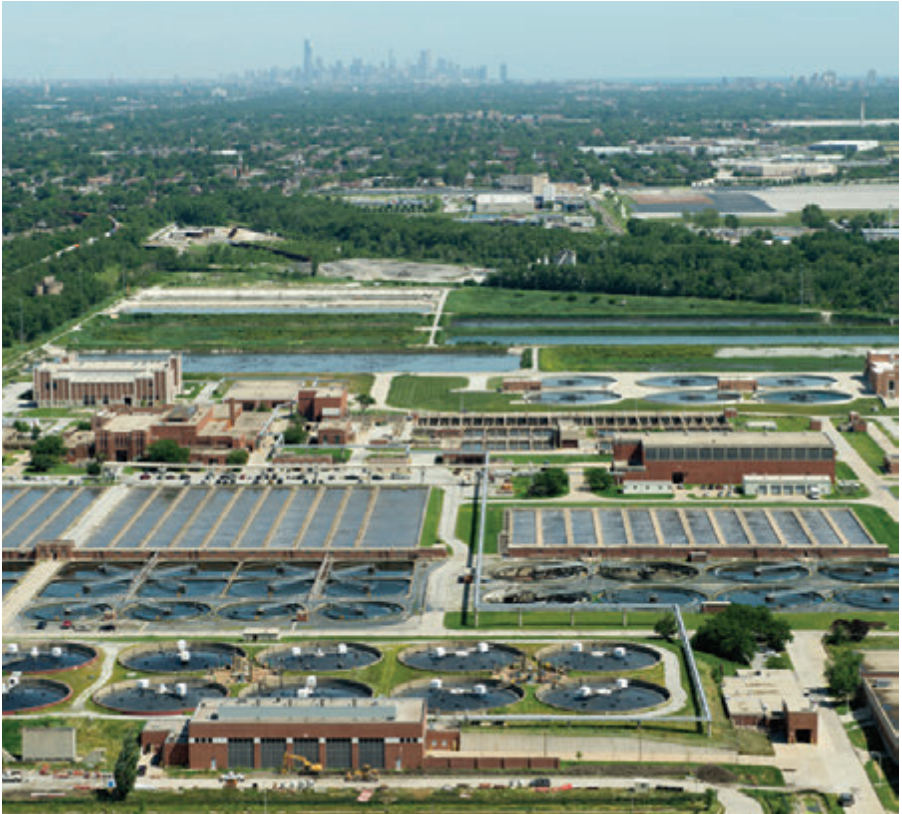
The disinfection facility at the Calumet Water Reclamation Plant was completed and put into operation in 2015.
