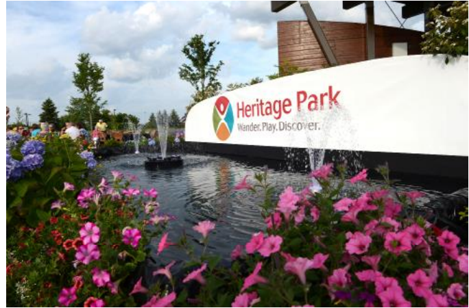
The MWRD joined the Wheeling Park District and Village of Wheeling in opening the Heritage Park Flood Control Facility in Wheeling. The facility is situated in the Des Plaines River watershed near the intersection of Dundee and Wolf Roads in Wheeling. The complex provides compensatory floodwater storage upstream of the U.S. Army Corps of Engineers' Levee 37 flood control structure in Mount Prospect and Prospect Heights.
