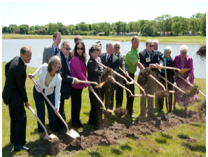
Commissioners Terrence J. O'Brien, Debra Shore and Mariyana T. Spyropoulos were joined by federal, state and local leaders to break ground on the Heritage Park Flood Control Facility in Wheeling, IL.
