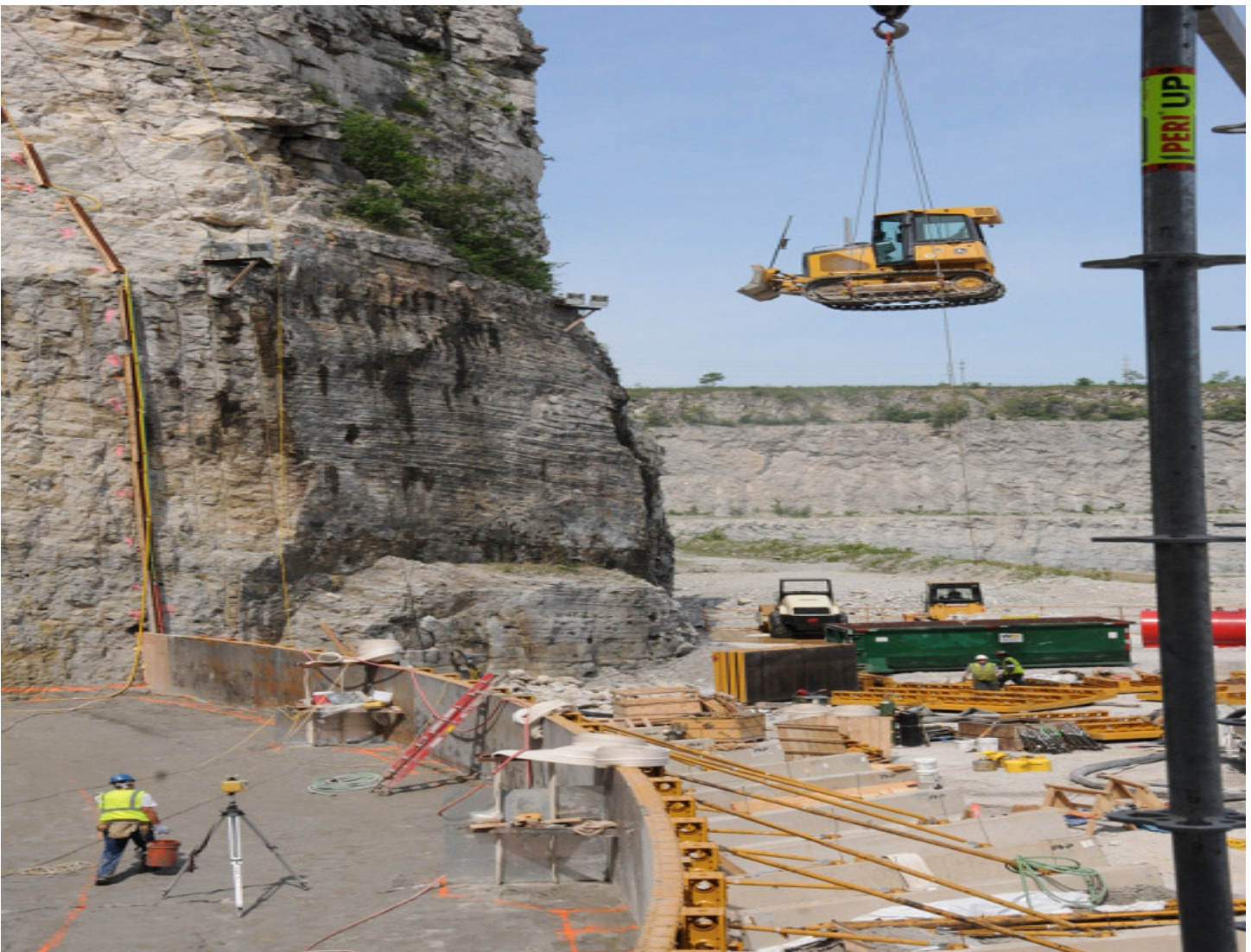
The Thornton Reservoir Dam stands at a height of 112 feet and its construction required 32,000 cubic yards of concrete.
