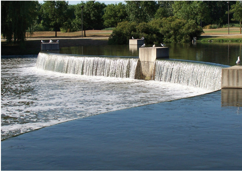
SEPA stations are not only beautiful, but also provide habitat for the abundant wildlife. The cascading waterfalls are environmentally friendly and provide vital oxygen to the waterways.
