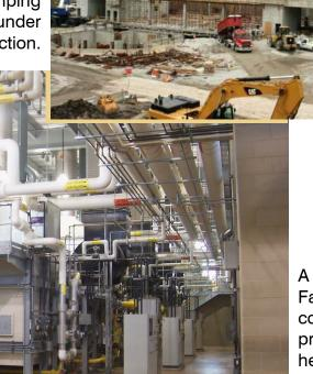
A new Central Boiler Facility has been constructed which will provide additional heating requirements with high efficiency boilers which will maximize digester gas usage.
