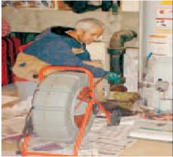
Locating the pipe
