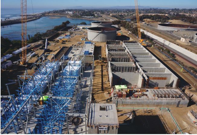
Water desalination plant construction in Carlsbad, CA
